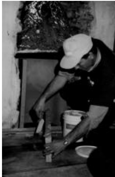
The shiplap edge of the flare is buttered with Super Cement®. The back side of the flare should be insulated with Cera-Foil.
