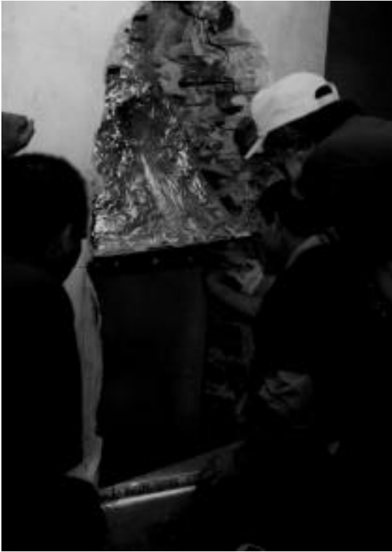
The shiplap edge of the flare is buttered with Super Cement®. The back side of the flare should be insulated with Cera-Foil.
