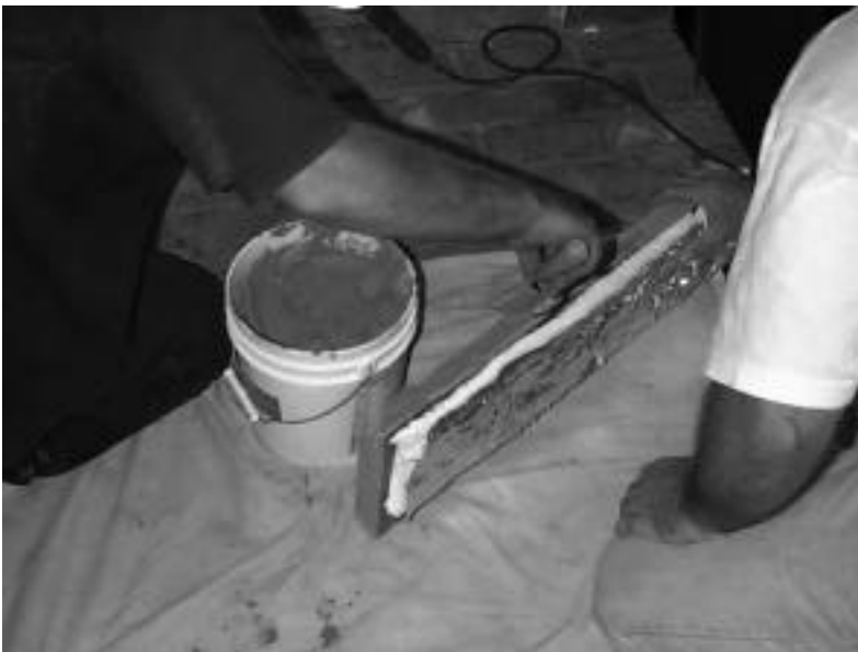
The shiplap edge of the flare is buttered with Super Cement®. The back side of the flare should be insulated with Cera-Foil.
